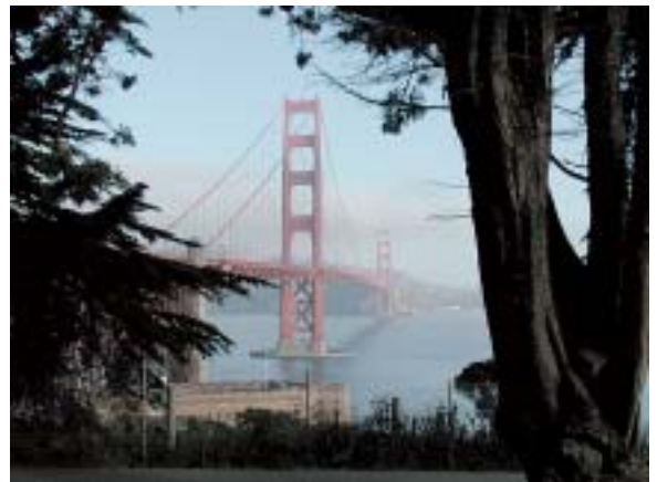
Golden Gate Bridge
